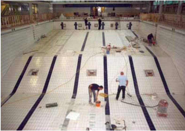
Removal of Defective Screeding
