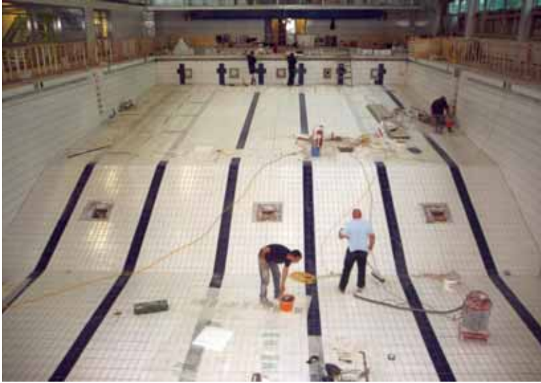
Removal of Defective Screeding
